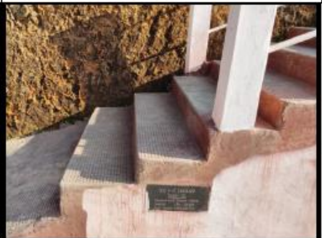
Photo : Construction of Steps at Sailulak
