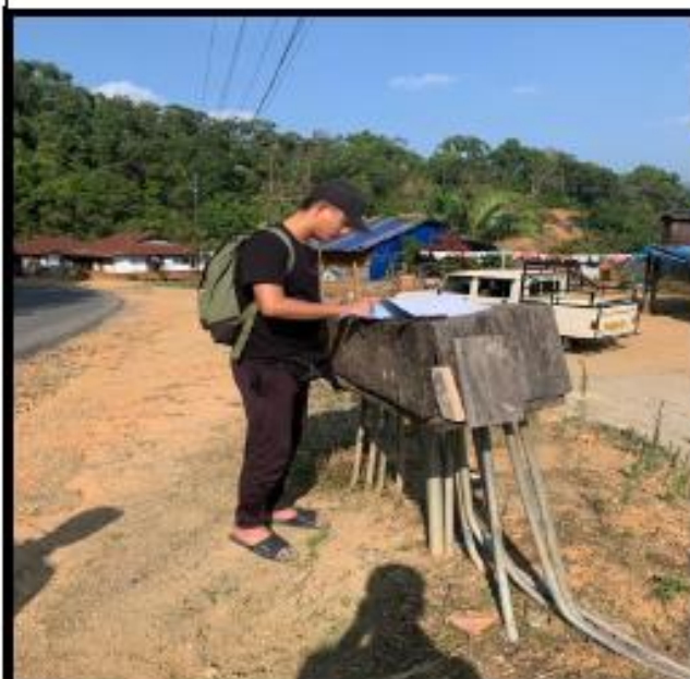
Photo : Construction of Water Pipeline at Zyhno B
