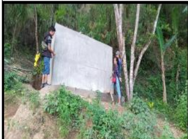
Photo : Construction of Rain Water Harvesting Tank at Cherhlun
