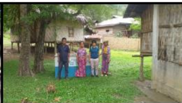
Photo : Construction of Compost pit at Kiasie
