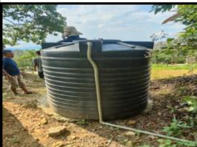
Photo : Providing & Fitting 20mm G-Pipe at Khuangleng
