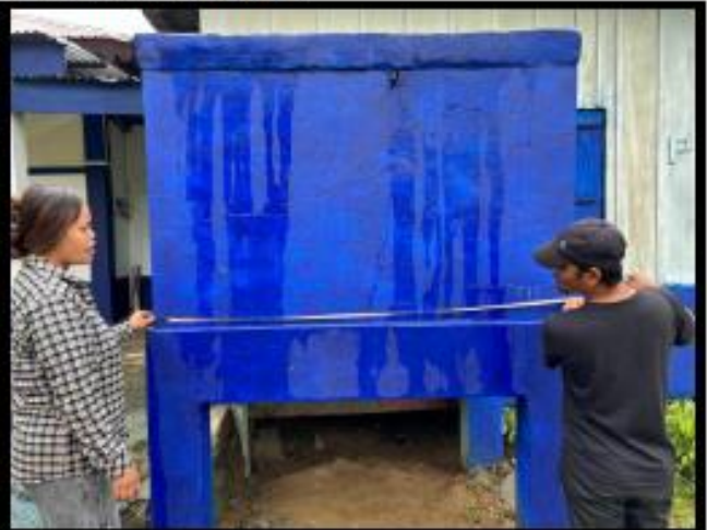
Photo : Construction of Ferro-cement water tank
