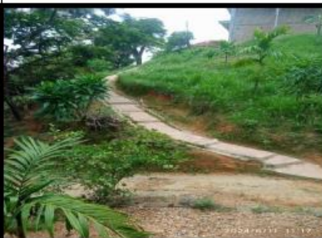
Photo : Construction of PCC steps with chequered tile at Chithar
