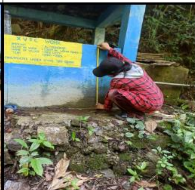
Photo : Construction of Water Tank at New Laty
