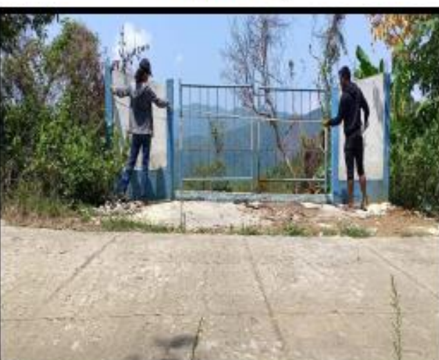
Photo : Construction of Dumping Ground
