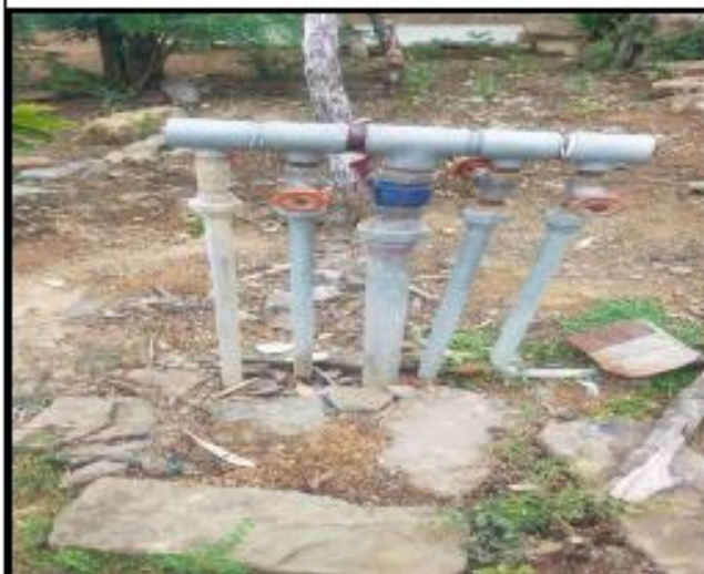
Photo : Construction of T-Cluster at III. HNAHTHIAI DISTRICT
