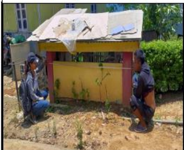
Photo : Construction of Water Tank
