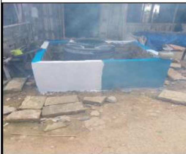
Photo : Construction of Water Reservoir at Tuichawngtlang
