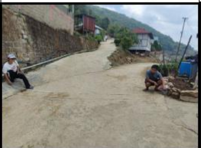
Photo : Construction of PCC Flooring/Land leveling
