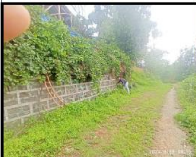
Photo : Construction of retaining wall
