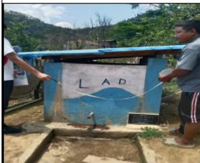
Photo : Construction RCC Intake
