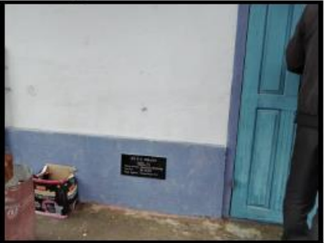
Photo : Repairing of BNRGSK Hall at Lungchhuan
