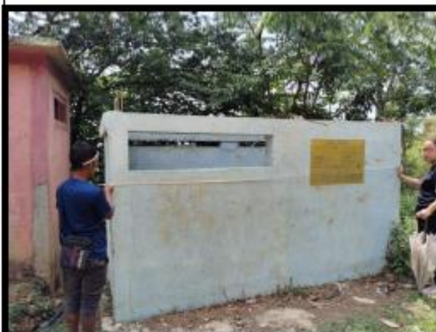
Photo : Construction of Waste Collection at Tipa D-II
