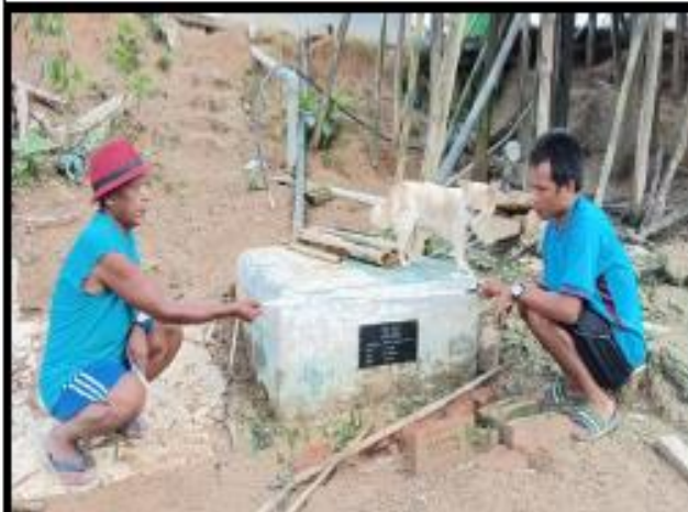
Photo : Construction of Community Soak Pit at Mautlang
