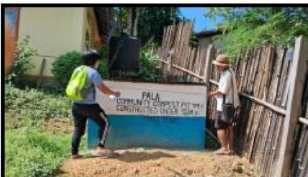
Photo : Construction of Community Compost Pit at Pala
