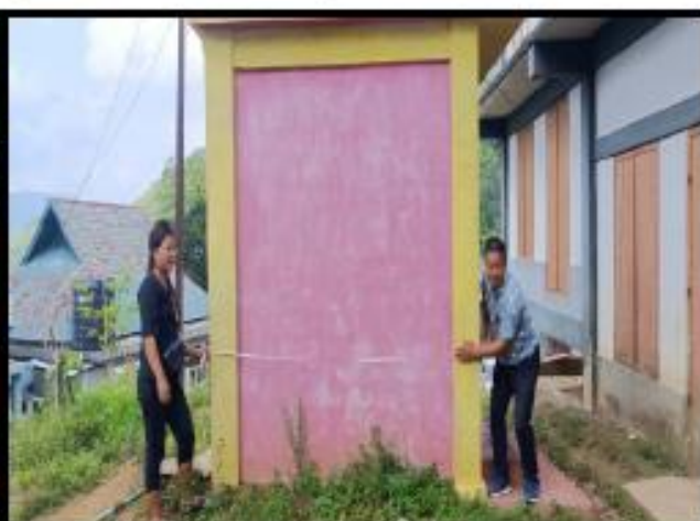
Photo : Construction of Public Bathroom at Pangzawl N
