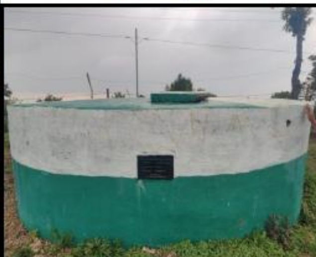
Photo : Construction of RCC Reservoir at Khuangleng
