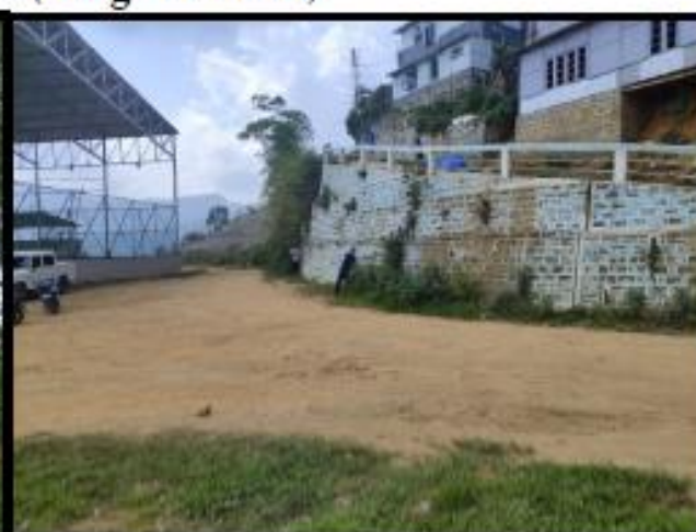
Photo : Construction of retaining wall & Hand railing near Ramthar GSA Field
