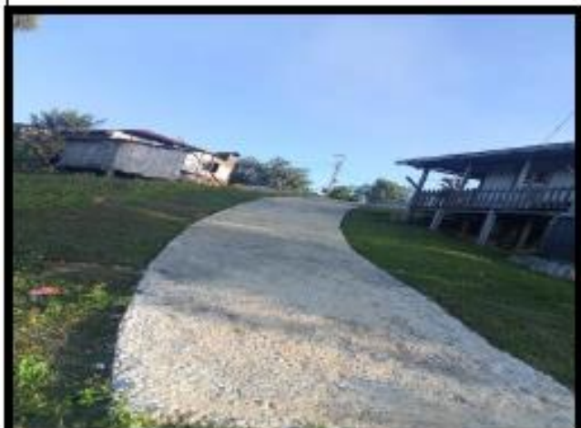
Photo : Construction of PCC pavement at Thangte
