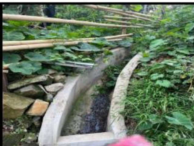
Photo : Construction of Side drain at Hmar Veng
