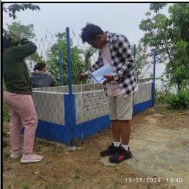
Photo : Construction of Compost pit, Lungtan
