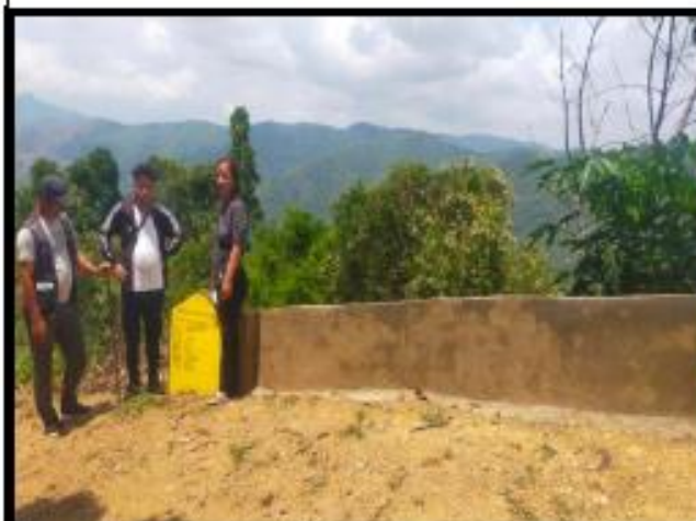
Photo : Construction of Dumping Ground at Zawngtetui
