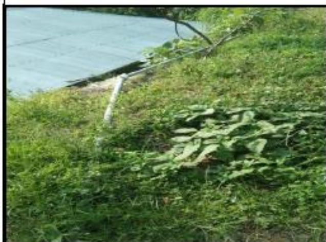
Photo : Extention of distribution line with T- cluster at Gosen Veng
