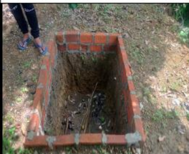
Photo : Construction of Compost Pit
