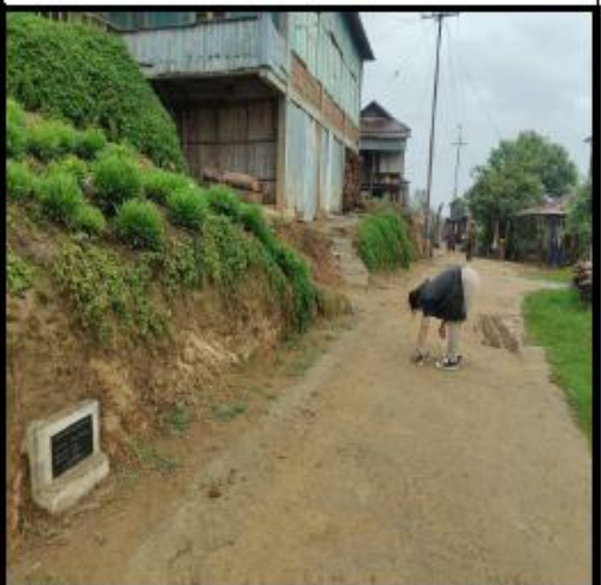
Photo : Auditor in action (Measuring PCC Flooring)
