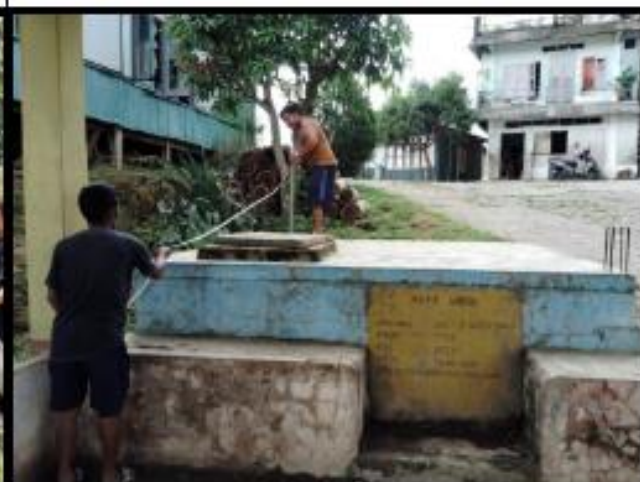
Photo : Construction of Water Tank at Saikou B
