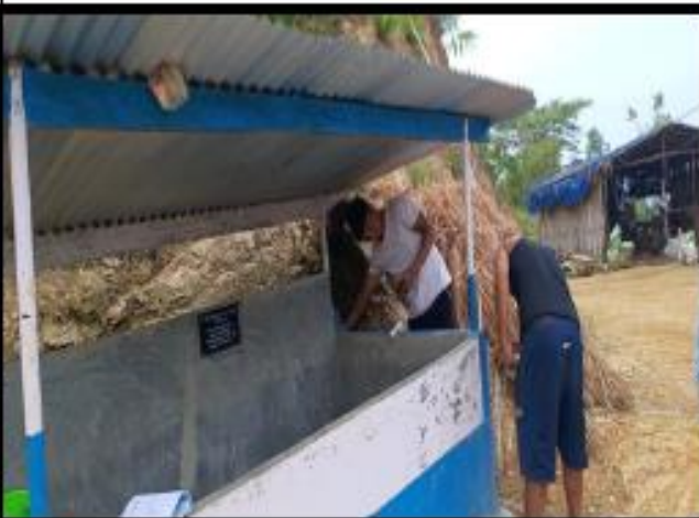
Photo : Construction of Water Tanky at Ngharchhip
