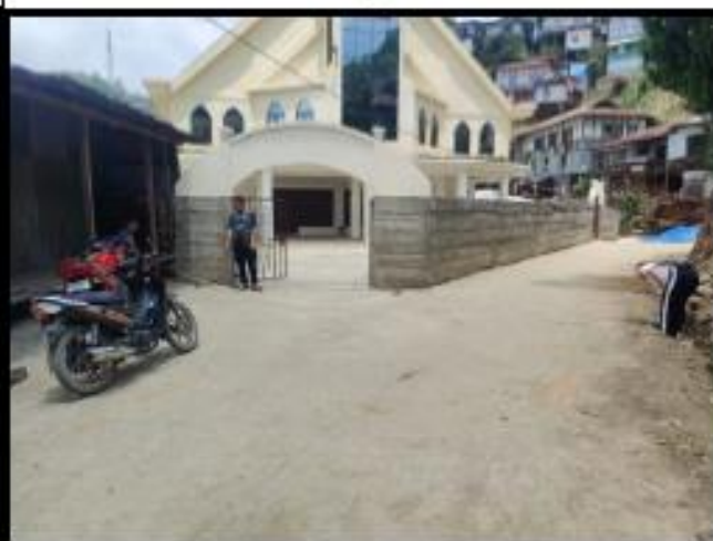
Photo : Construction of PCC white topping Pu Bualthanga's house to IKK church at Vaphai
