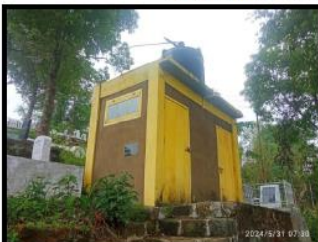
Photo : Construction of Public Urinal and Toilet at Thlanmual No. 1 at Zotlang
