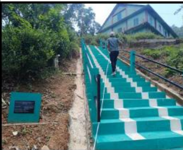
Photo : Construction of RCC Step at Pawlrang
