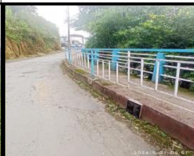
Photo : Construction of foot-path with hand railing
