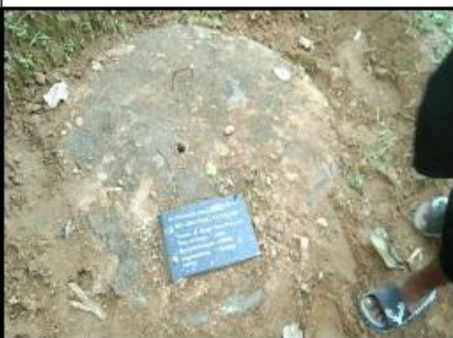
Photo : Construction of Single pit to Twin pit at Saiphai
