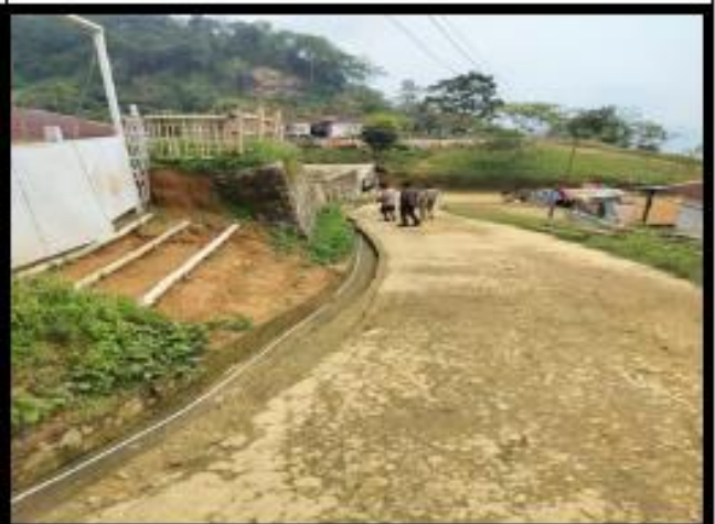
Photo : Construction of Side drain
