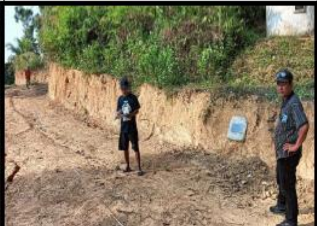
Photo : Construction of Village internal road at Hmunnuam
