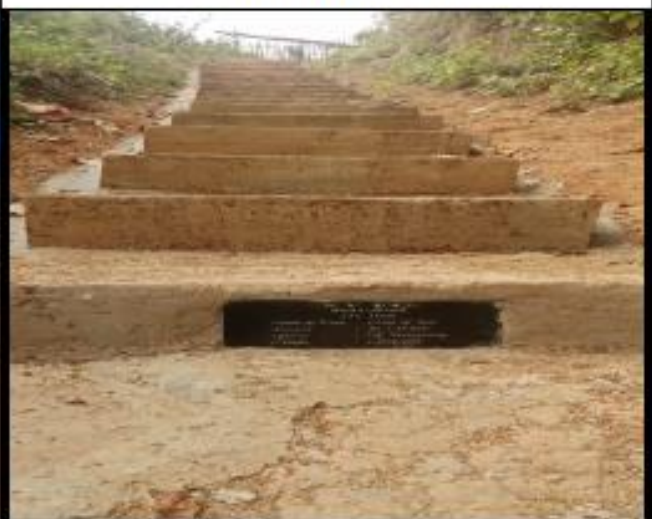
Photo : Construction of Steps at Tuisentlang
