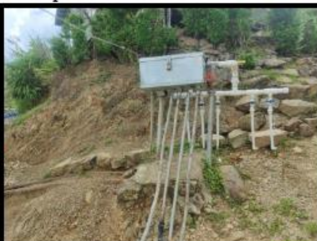
Photo : Construction of T-Cluster at Sesih
